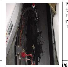
Mount rule pump after gate valve near battery. Use Teflon tape on the <sup>3</sup>/<sub>4</sub> male to <sup>3</sup>/<sub>4</sub> female PVC fitting. Clear braided hose or supplied poly hose. Heating hose might be necessary to install on fitting. Install threaded fitting with Teflon tape.
